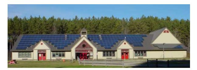
In November of 2013, the Ripton Elementary School brought a 50 kW solar array on line to provide 75 percent of the school's energy through the year. 198 panels sit on a new, standing-seam metal roof, gathering sunlight and serving as a model for future projects. This clean, renewable system is expected to begin paying for itself by the third year of operation, producing 54.1MWh of power in 2014 even under below average sun exposure.
