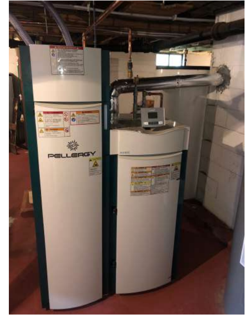
Hydronic Heaters (aka Boilers)
