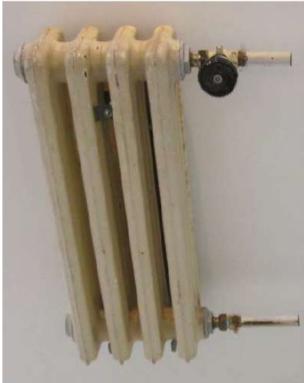
Traditional cast-iron radiator
