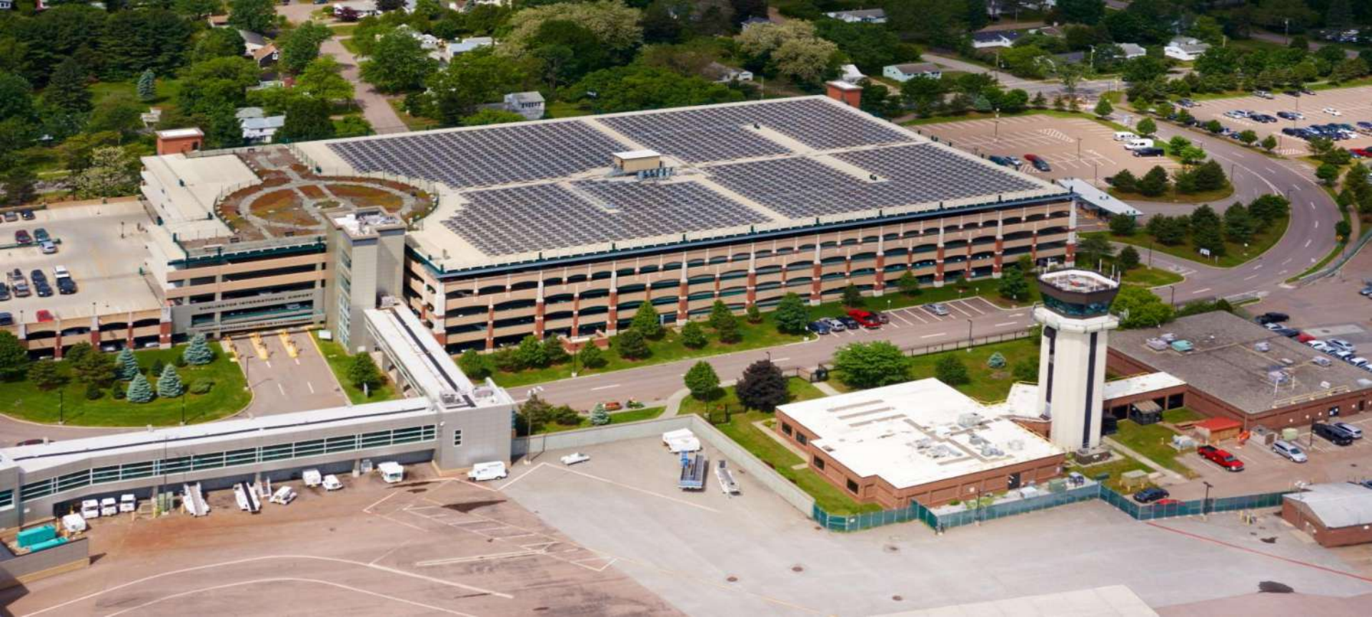
Photo: Encore's Burlington Airport project
