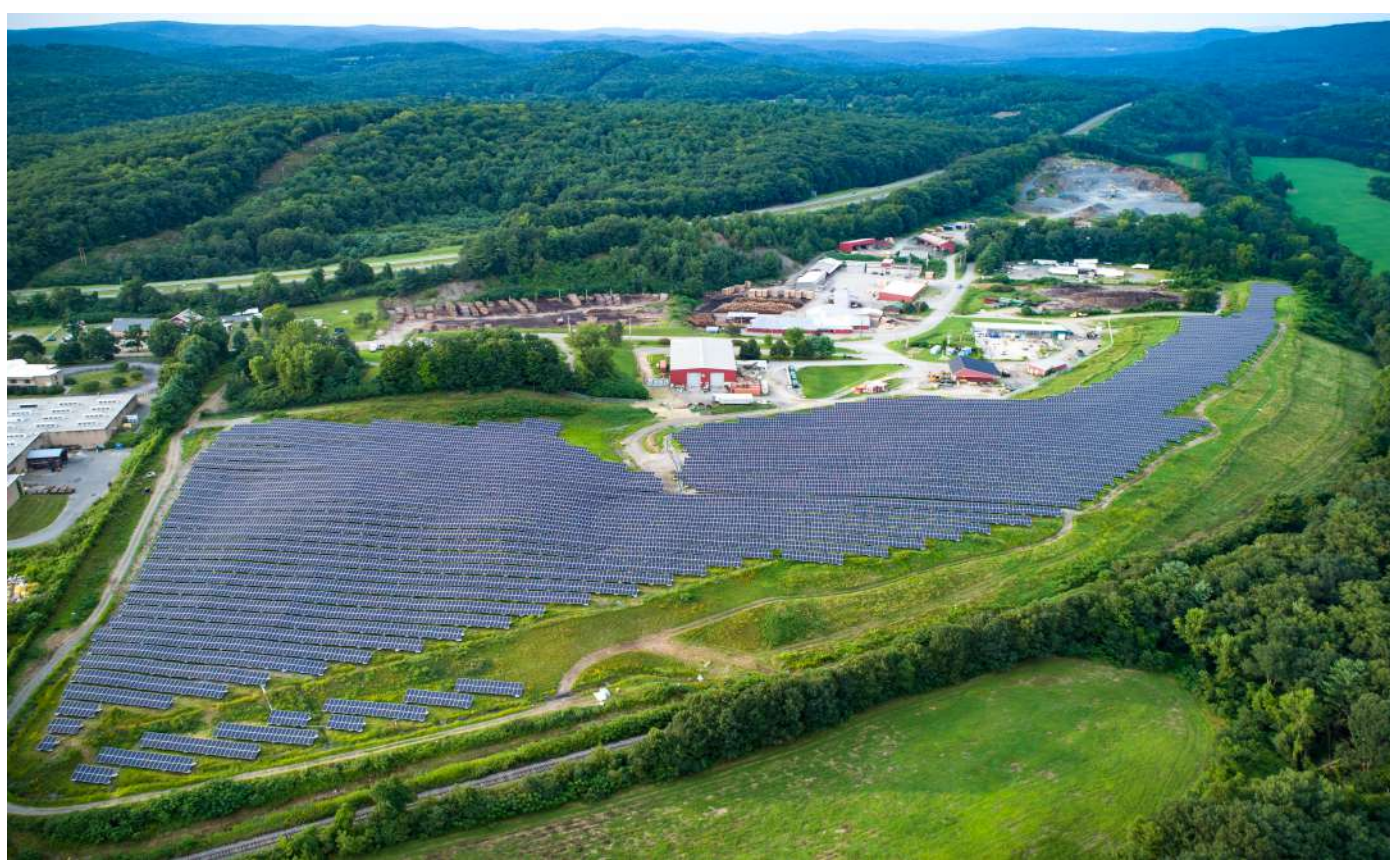
Photo: Encore's 5MW Brattleboro, VT Landfill Solar Project
