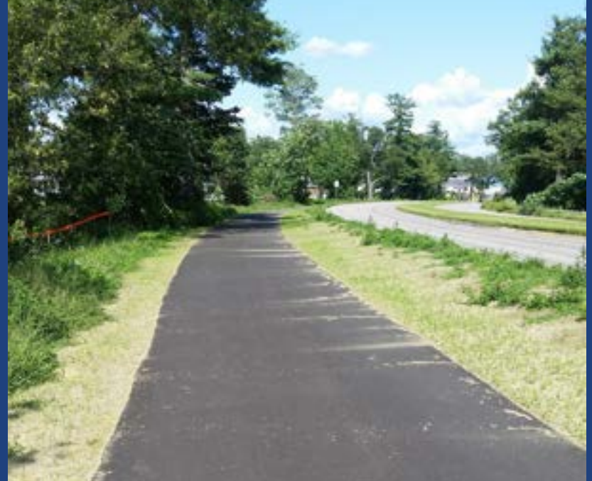
Shared use path being built along Route 15 in Colchester
